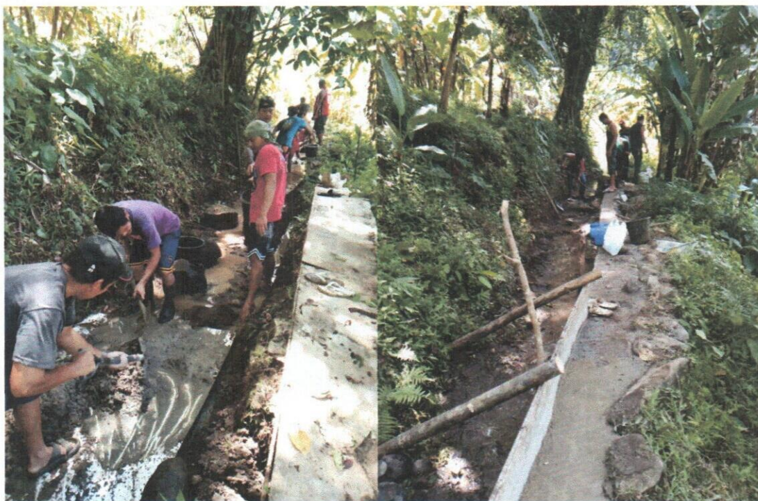
Waterwheel Canal Repair
