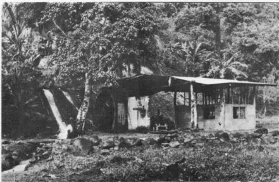
The old VISCA waterwheel is being restored to run the abaca stripping machine and to generate electricity.
