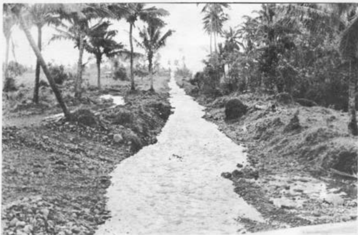
The Calbiga-a river has been straightened to minimize destruction of experimental fields during floods.
